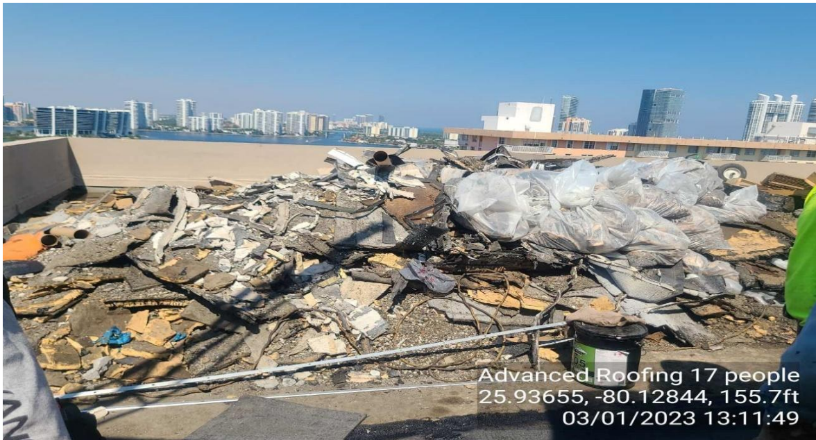
Advanced Roofing east 25.93664, -80.12777, 124.9ft 03/15/2023 09:52:44
