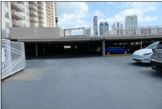
Photo 47 Building Structure and Envelope
