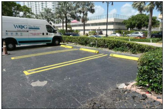
Photo 282 Site and Building Improvements
