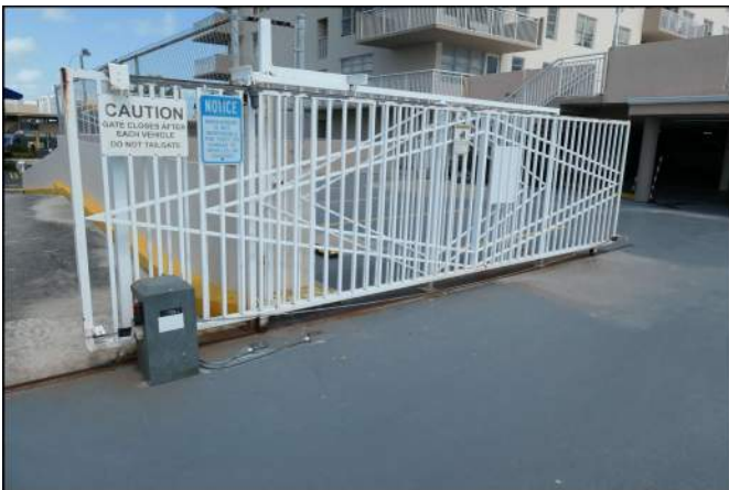
Photo 275 Site and Building Improvements
