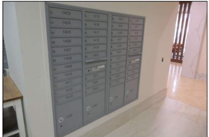
Photo 262 Site and Building Improvements
