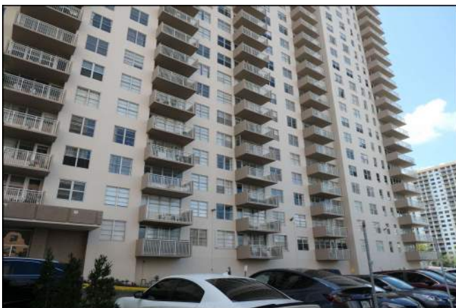
Photo 11 Building Structure and Envelope
