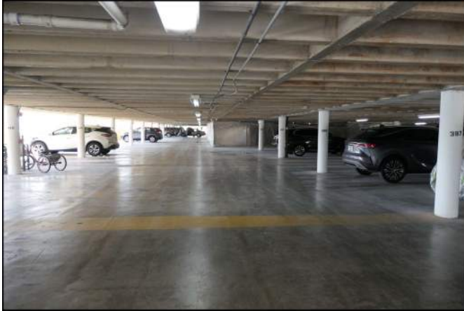
Photo 43 Building Structure and Envelope
