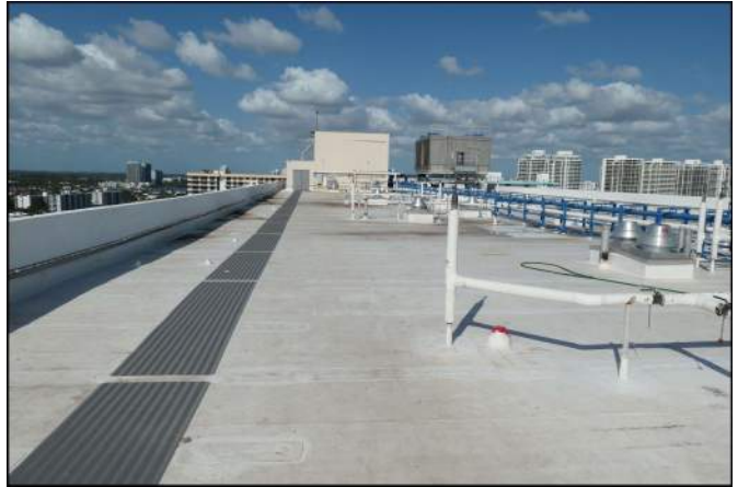
Photo 16 Building Structure and Envelope
