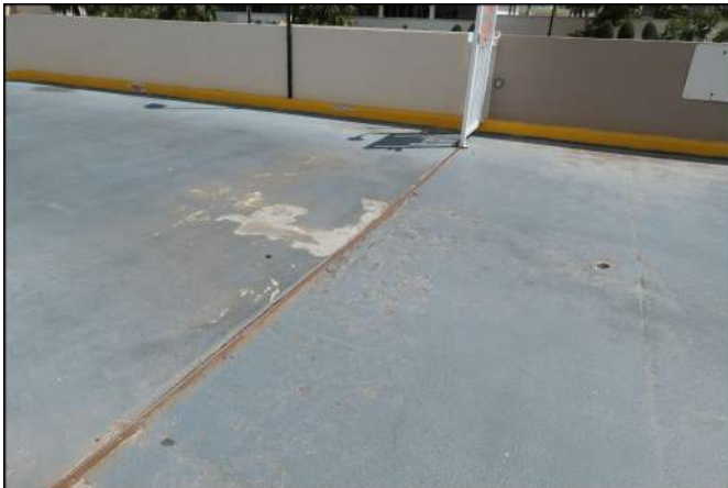
Photo 45 Building Structure and Envelope
