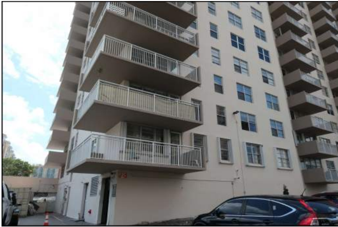
Photo 03 Building Structure and Envelope
