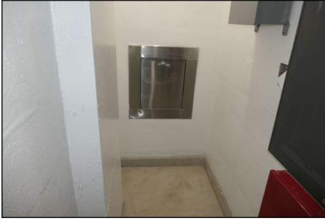
Photo 265 Site and Building Improvements
