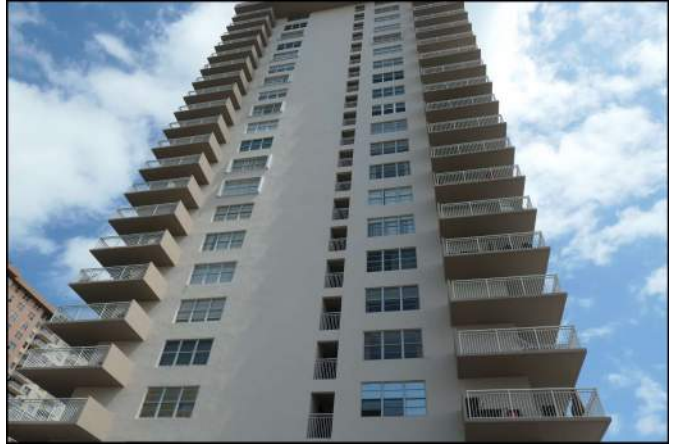
Photo 14 Building Structure and Envelope
