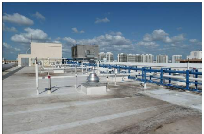
Photo 18 Building Structure and Envelope
