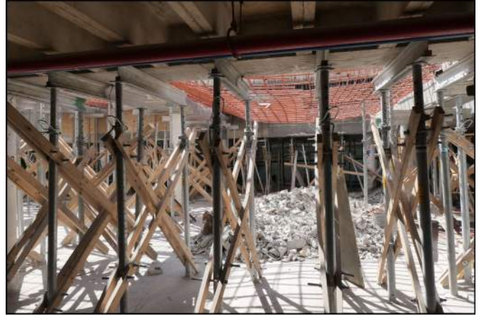
Photo 38 Building Structure and Envelope
