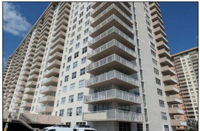
Photo 06 Building Structure and Envelope
