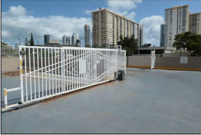
Photo 271 Site and Building Improvements
