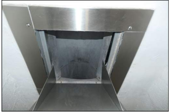
Photo 266 Site and Building Improvements
