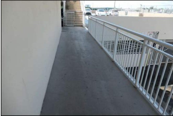
Photo 25 Building Structure and Envelope
