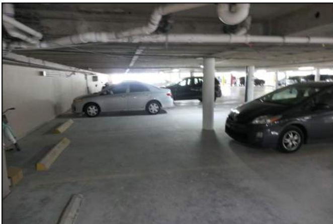
Photo 41 Building Structure and Envelope
