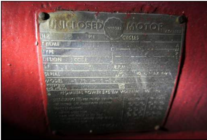
Photo 99 Fire Protection Systems
