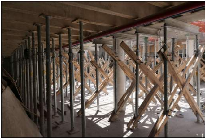
Photo 39 Building Structure and Envelope
