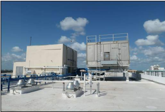
Photo 21 Building Structure and Envelope
