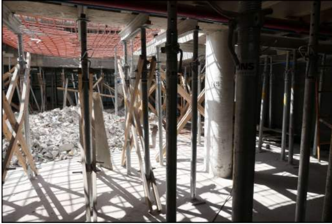
Photo 37 Building Structure and Envelope
