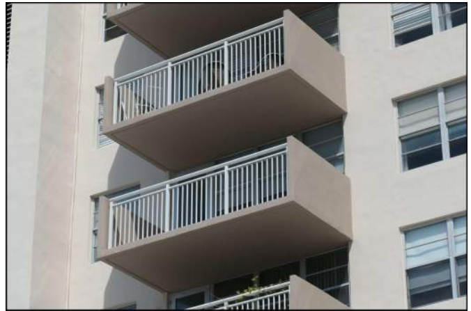
Photo 10 Building Structure and Envelope
