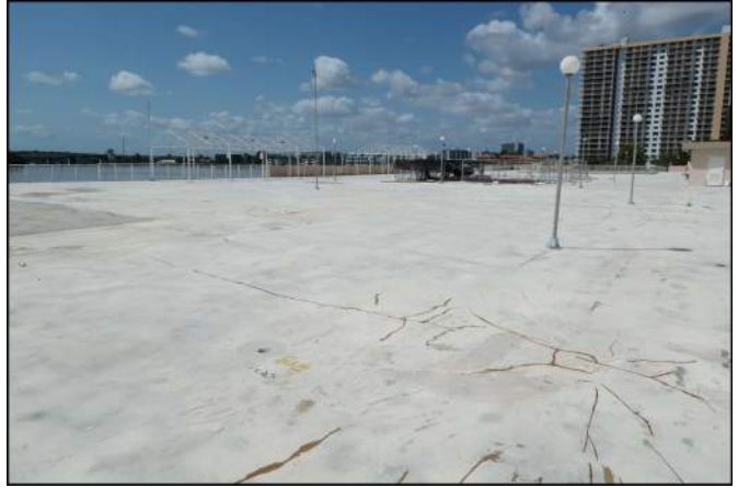
Photo 32 Building Structure and Envelope
