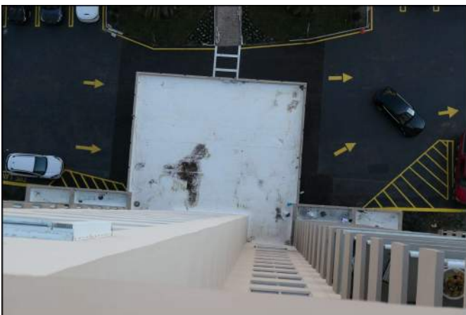
Photo 23 Building Structure and Envelope
