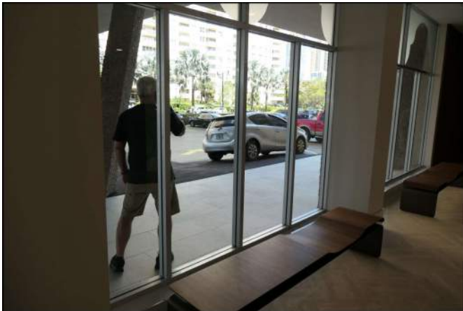
Photo 27 Building Structure and Envelope
