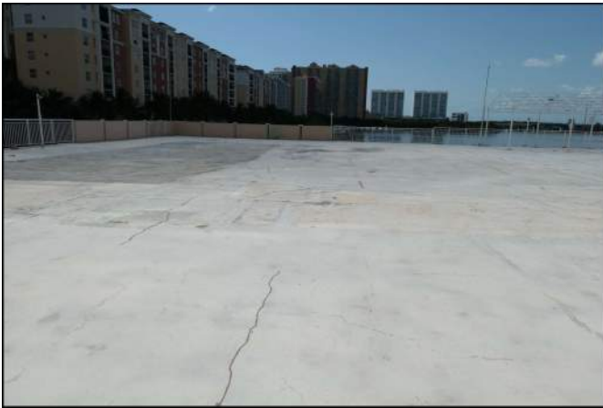
Photo 33 Building Structure and Envelope
