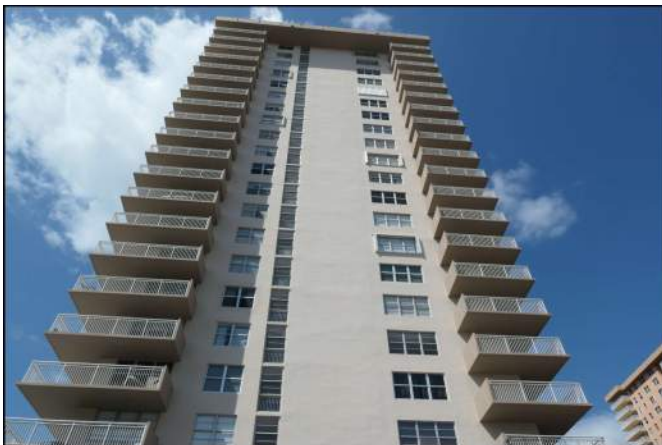
Photo 05 Building Structure and Envelope
