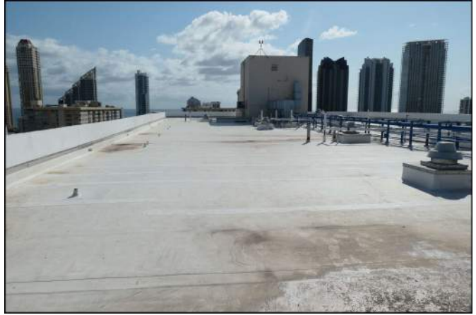
Photo 20 Building Structure and Envelope
