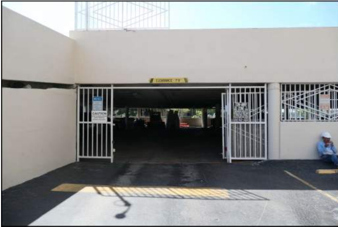
Photo 273 Site and Building Improvements
