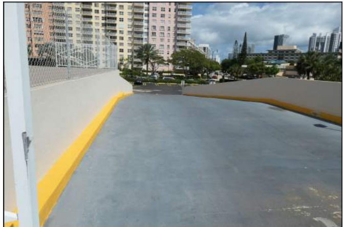
Photo 46 Building Structure and Envelope
