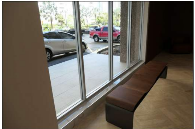
Photo 28 Building Structure and Envelope
