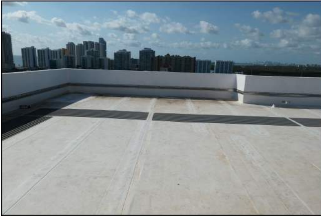
Photo 15 Building Structure and Envelope
