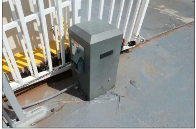
Photo 272 Site and Building Improvements
