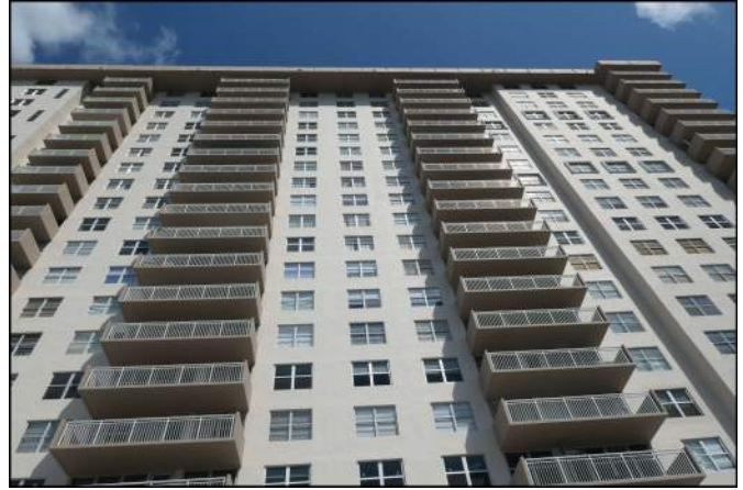
Photo 08 Building Structure and Envelope
