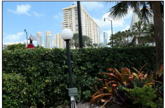
Photo 286 Site and Building Improvements
