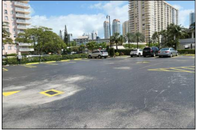
Photo 278 Site and Building Improvements
