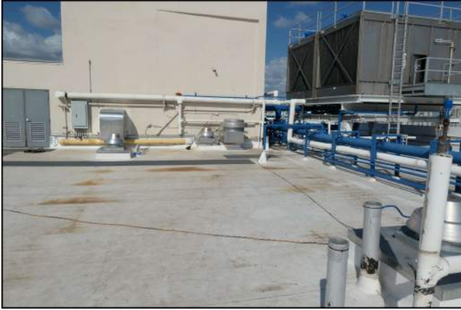
Photo 19 Building Structure and Envelope
