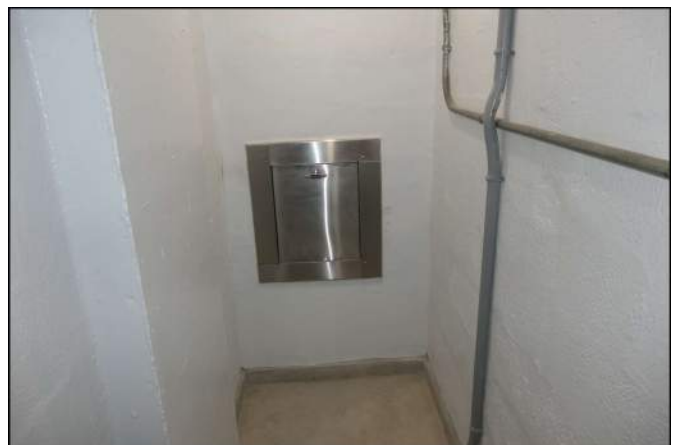
Photo 264 Site and Building Improvements
