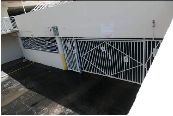
Photo 277 Site and Building Improvements
