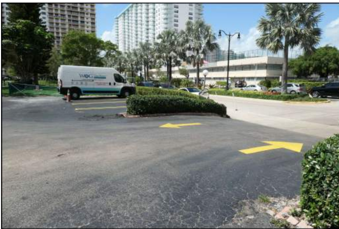
Photo 281 Site and Building Improvements
