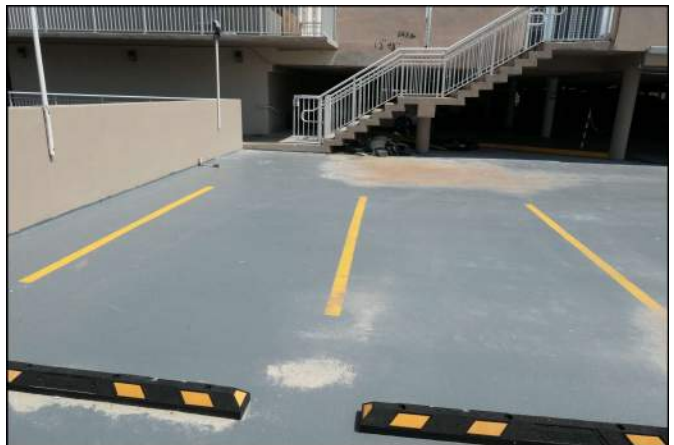
Photo 48 Building Structure and Envelope
