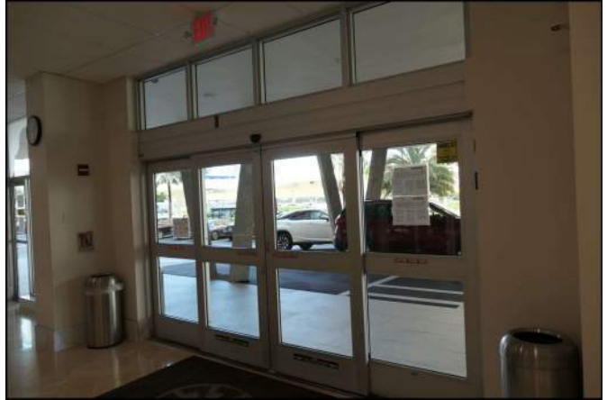
Photo 26 Building Structure and Envelope
