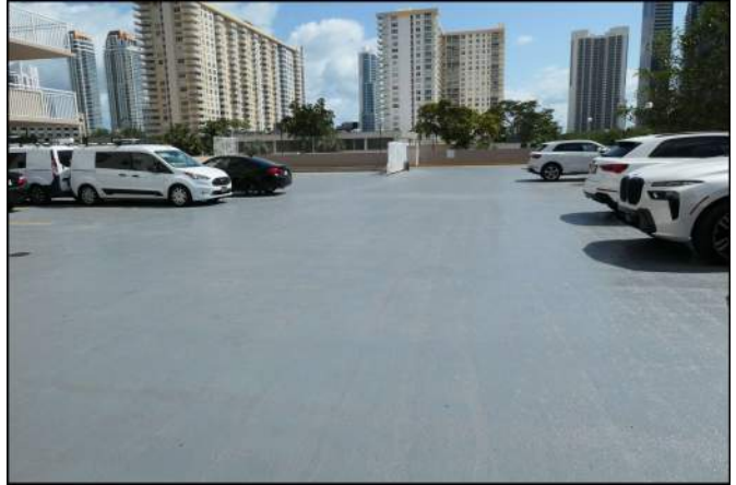
Photo 44 Building Structure and Envelope
