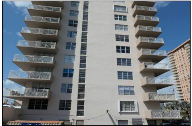
Photo 04 Building Structure and Envelope
