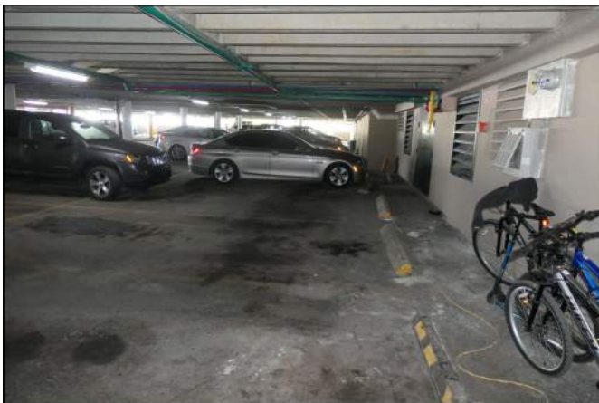
Photo 287 Site and Building Improvements
