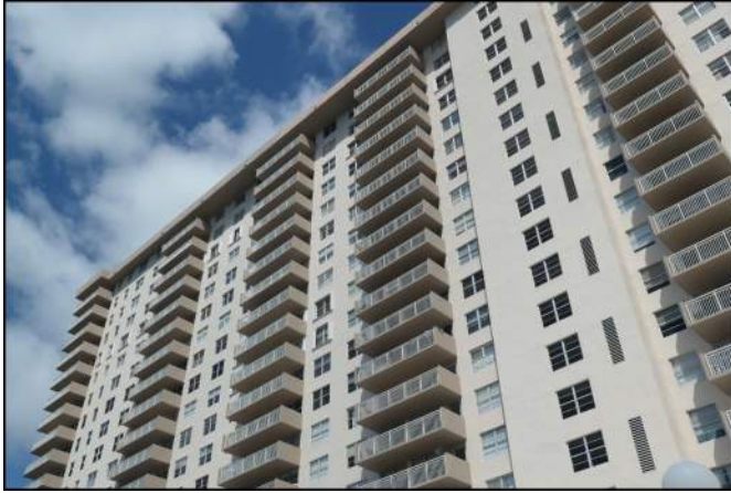
Photo 07 Building Structure and Envelope
