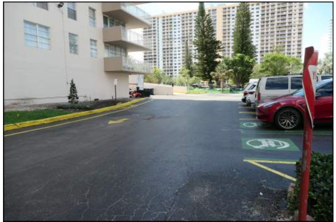
Photo 280 Site and Building Improvements
