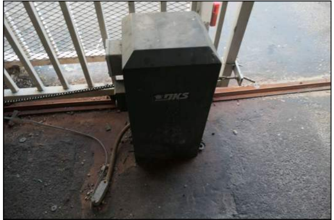
Photo 274 Site and Building Improvements
