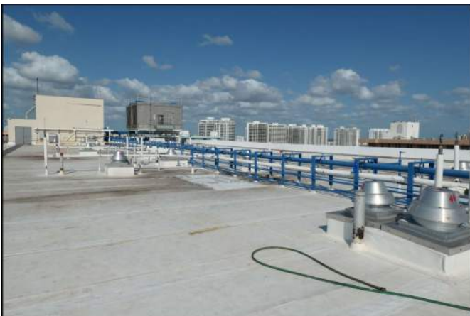
Photo 17 Building Structure and Envelope
