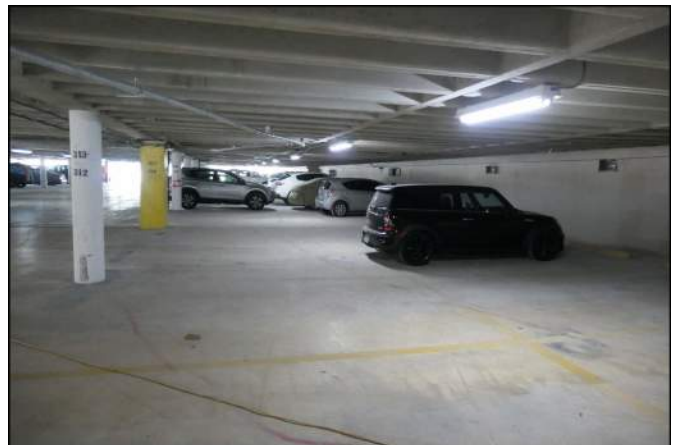
Photo 42 Building Structure and Envelope
