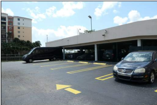
Photo 285 Site and Building Improvements
