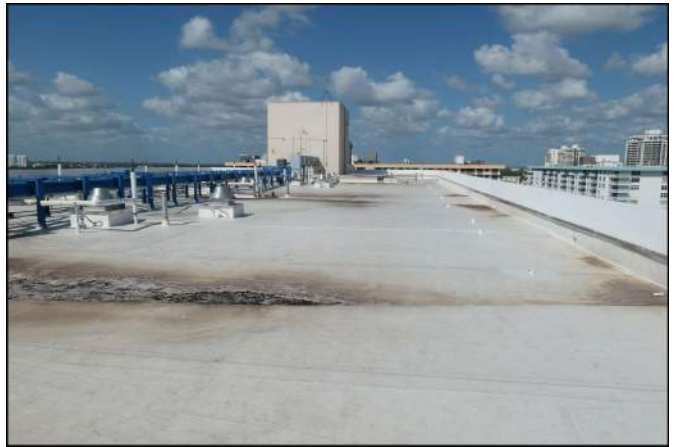
Photo 22 Building Structure and Envelope
