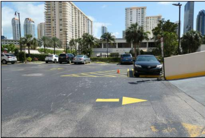
Photo 279 Site and Building Improvements
