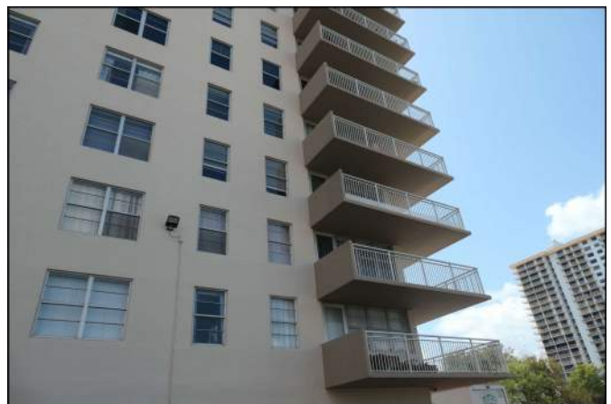
Photo 12 Building Structure and Envelope
