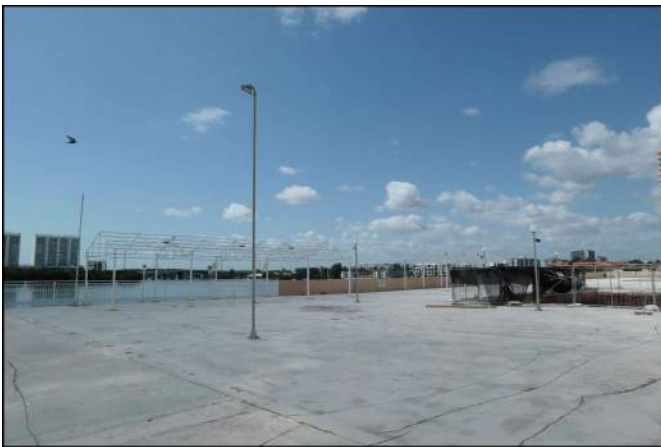
Photo 35 Building Structure and Envelope
