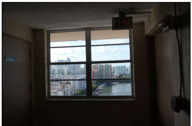
Photo 30 Building Structure and Envelope
