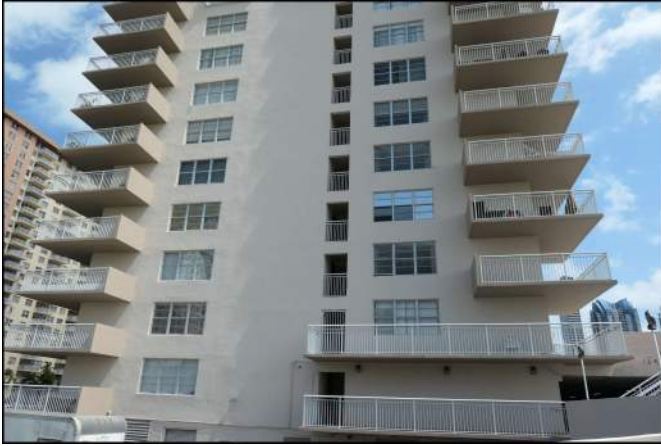
Photo 13 Building Structure and Envelope
