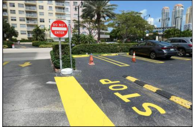
Photo 284 Site and Building Improvements
