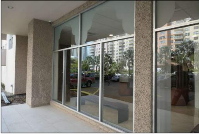
Photo 31 Building Structure and Envelope
