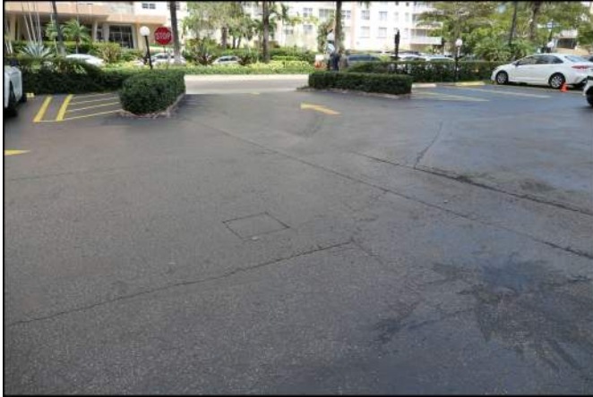
Photo 283 Site and Building Improvements
