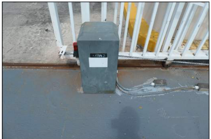
Photo 276 Site and Building Improvements
