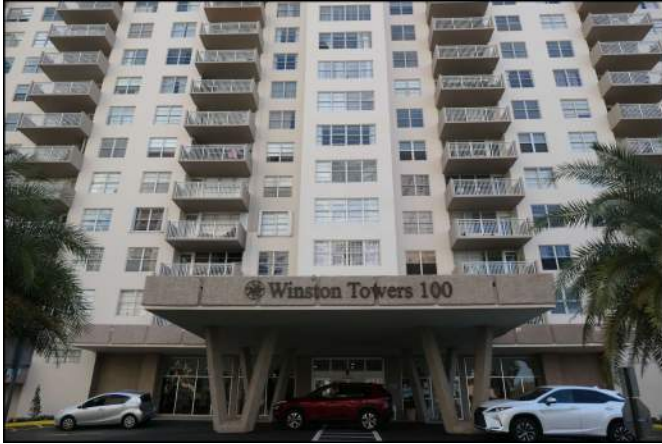
Photo 01 Building Structure and Envelope
