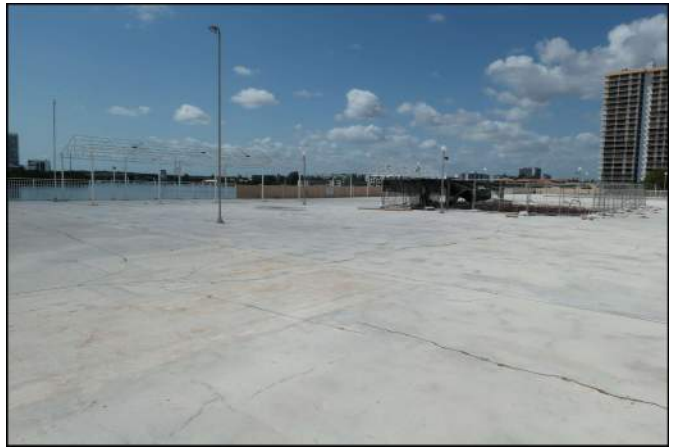
Photo 34 Building Structure and Envelope
