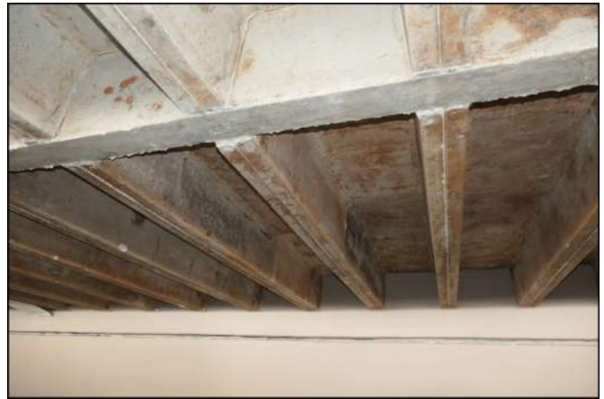
Photo 40 Building Structure and Envelope
