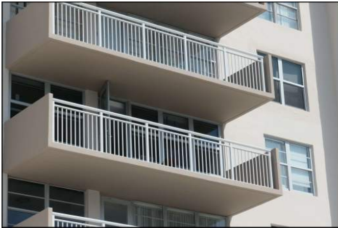
Photo 09 Building Structure and Envelope
