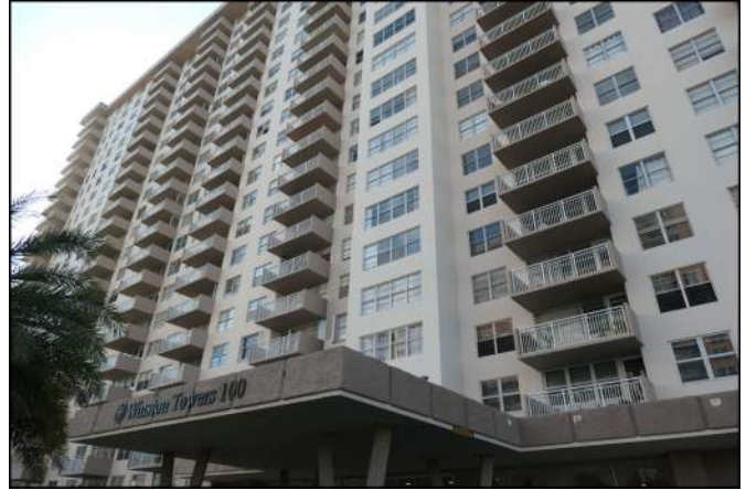
Photo 02 Building Structure and Envelope
