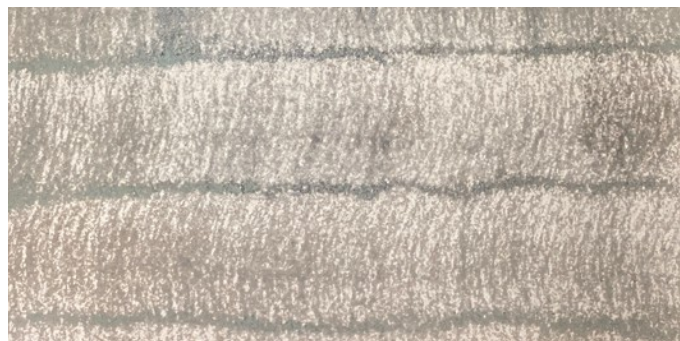
Proper Coverage on Insulation
