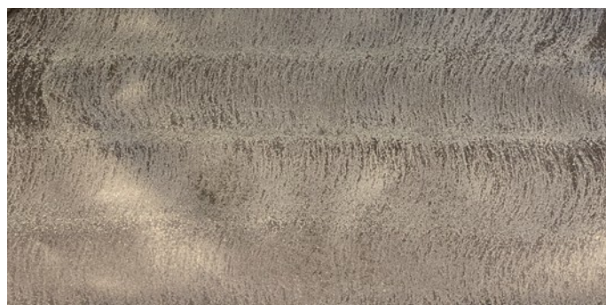
Proper Coverage on Membrane
