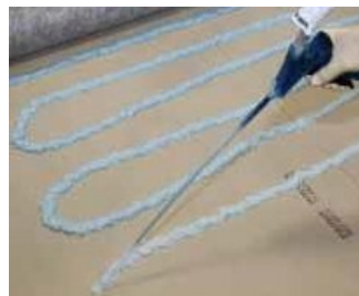
Apply using extension nozzle
